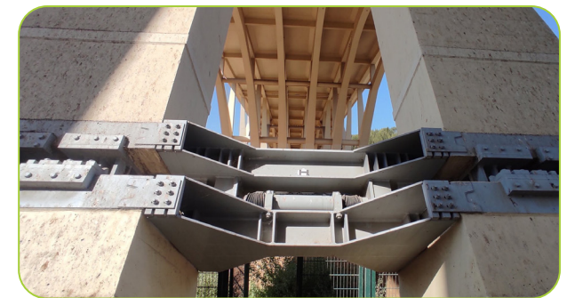
The base isolation and damping system
